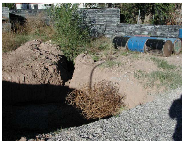
Figure 2. Cesspool under construction in Carlsbad
