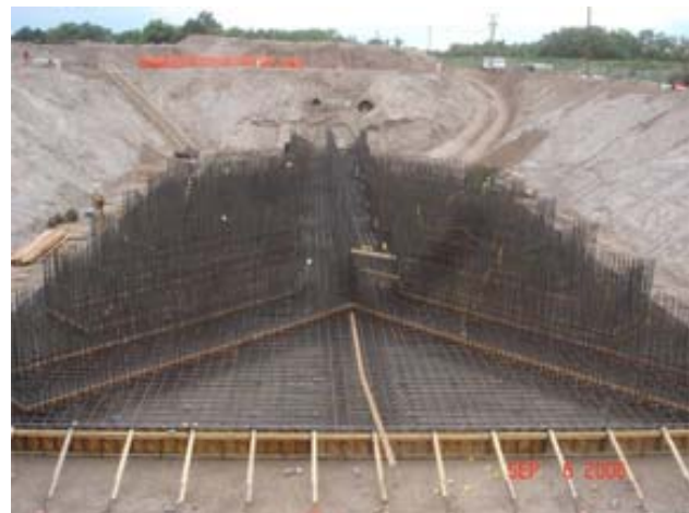
Figure 14. Raw water pump station wet well slab, rebar setting preparations
