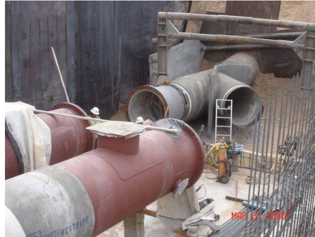
Figure 7. Rio Grande crossing, bottom of the west bluff 54-inch connection
