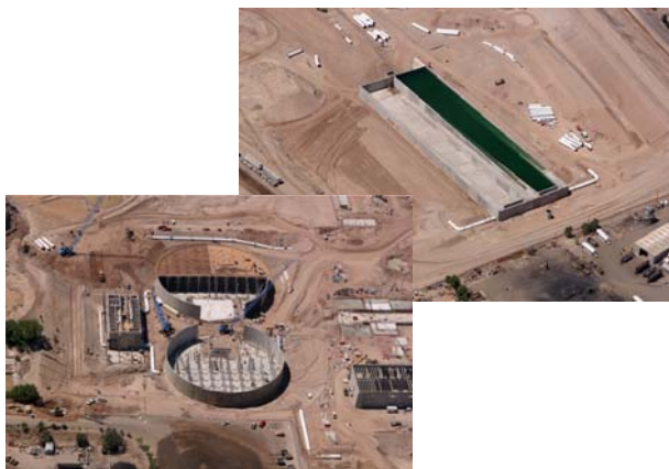
Figure 18. Aerial views of the tanks
