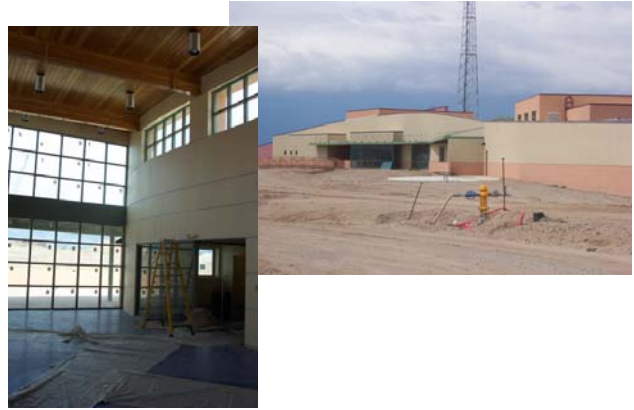
Figure 15. Completed administration building
