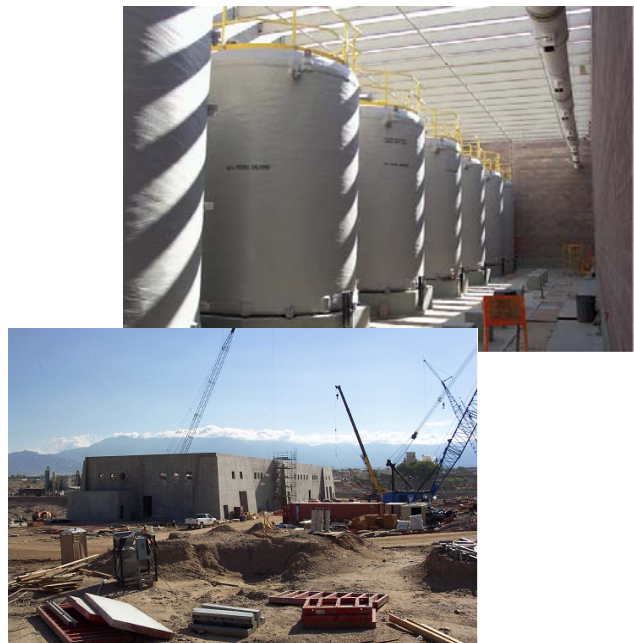
Figure 17. Chemical building onsite
