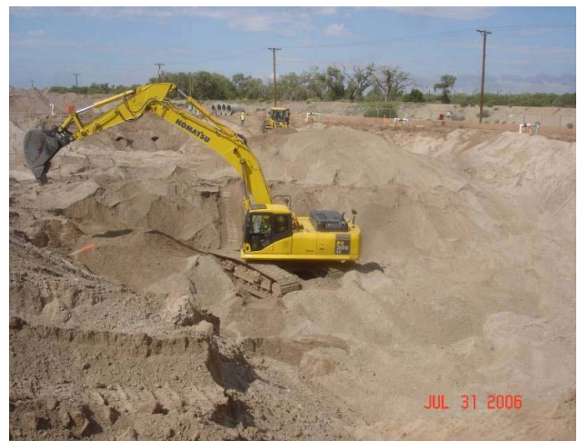
Figure 10. Excavation along Paseo del Norte
