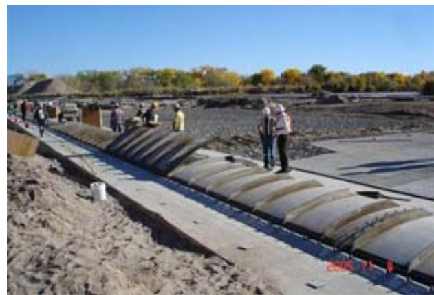
Figure 2. Diversion dam construction
