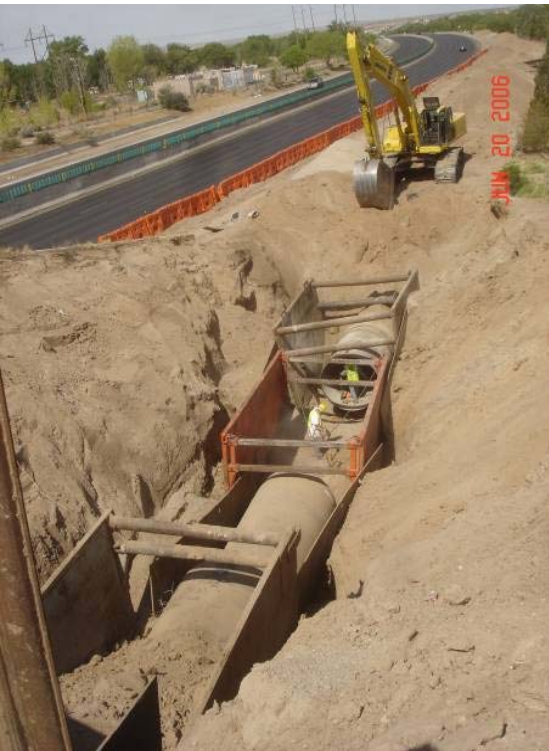
Figure 9. Raw water pipeline (72 inch) - looking west along Paseo del Norte
