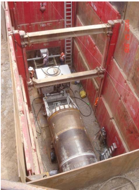
Figure 12. Bore pit at the south side of Carmony and Edith Blvd
